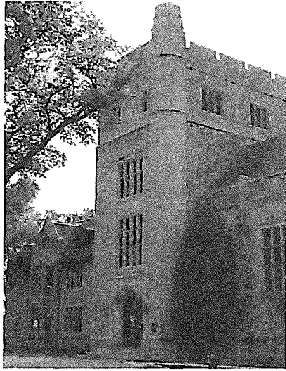
Main building on the north campus (500 Shaftesbury Boulevard) of Canadian Mennonite University Photo: CMU Communications Department
