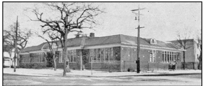
MBBC classroom and administration building, 1947 (29).
