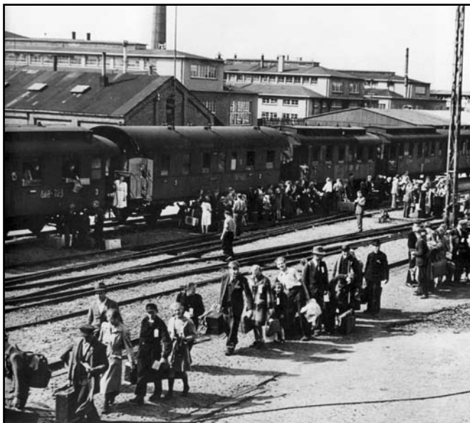
Mennonite refugees detrain in Bremen, Germany, en route to Canada, 1948 (67).
