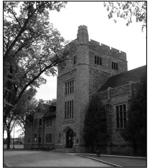
Canadian Mennonite University's (CMU) main administration and classroom building at 500 Shaftesbury Blvd. CMU brought together Canadian Mennonite Bible College, Concord College, and Menno Simons College in Christian university education (21).
