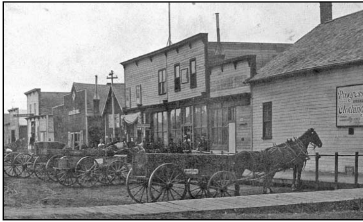
Looking south on Winkler's Main Street (48).
