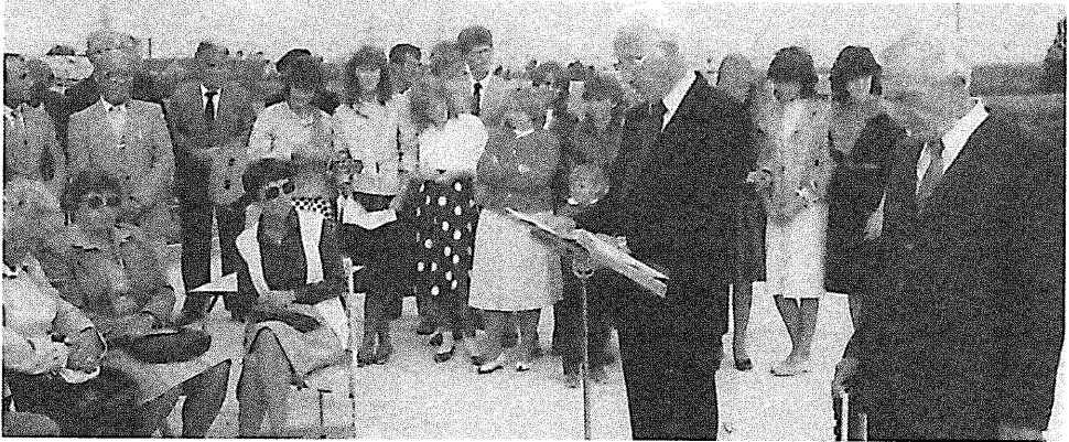
Ground breaking service for the new church building in Wolfsburg in 1983.
