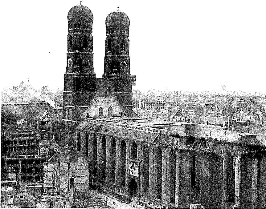
Heavily damaged Frauenkirche, München
