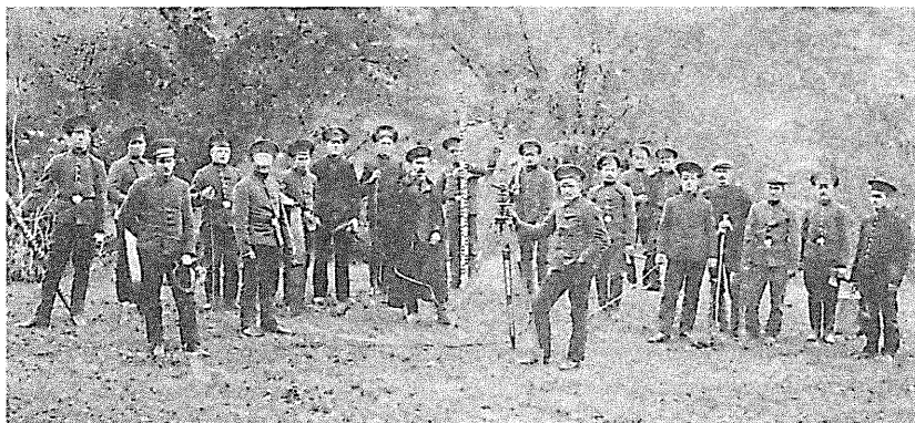
Mennonite men serving in the Forsteidienst help to build a road in the Crimea, ca. 1915. Jacob served in the forestry service for 22 months, first in the Alt-Berdian forest, then in the Crimea. Photo: MHCA
