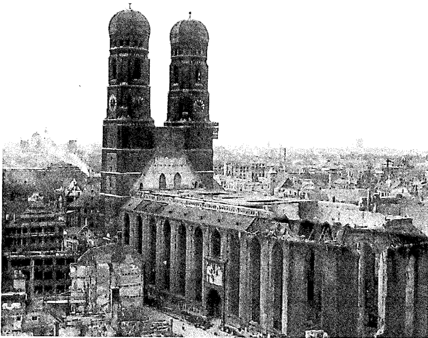
Heavily damaged Frauenkirche, München
