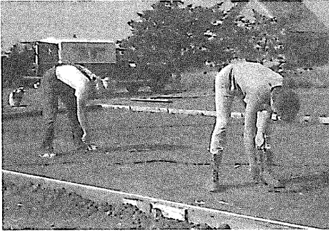
Voluntary Service workers repair the basketball court at the Hammon church.
