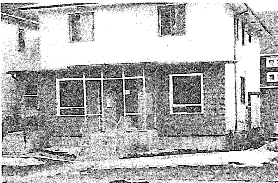
The Walnut Receiving Home at 171 Walnut Avenue in Winnipeg.
