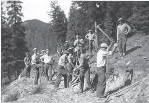
Mennonite conscientious objectors build a road in Jasper National Park, Alberta, 1941. Photo credit MHC.
