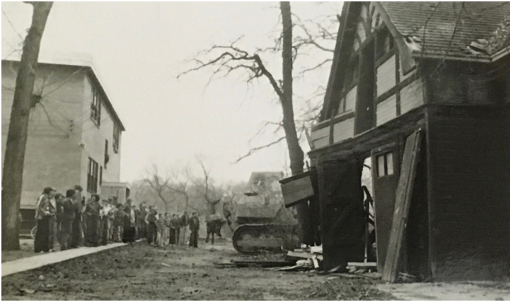
FIGURE 5.2. Demolition of the Art Barn
