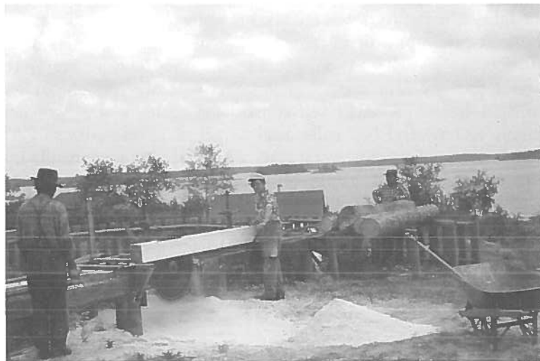
The sawmill which Mennonite Pioneer Mission flew in from southern Manitoba to produce dimensional lumber for log buildings.
